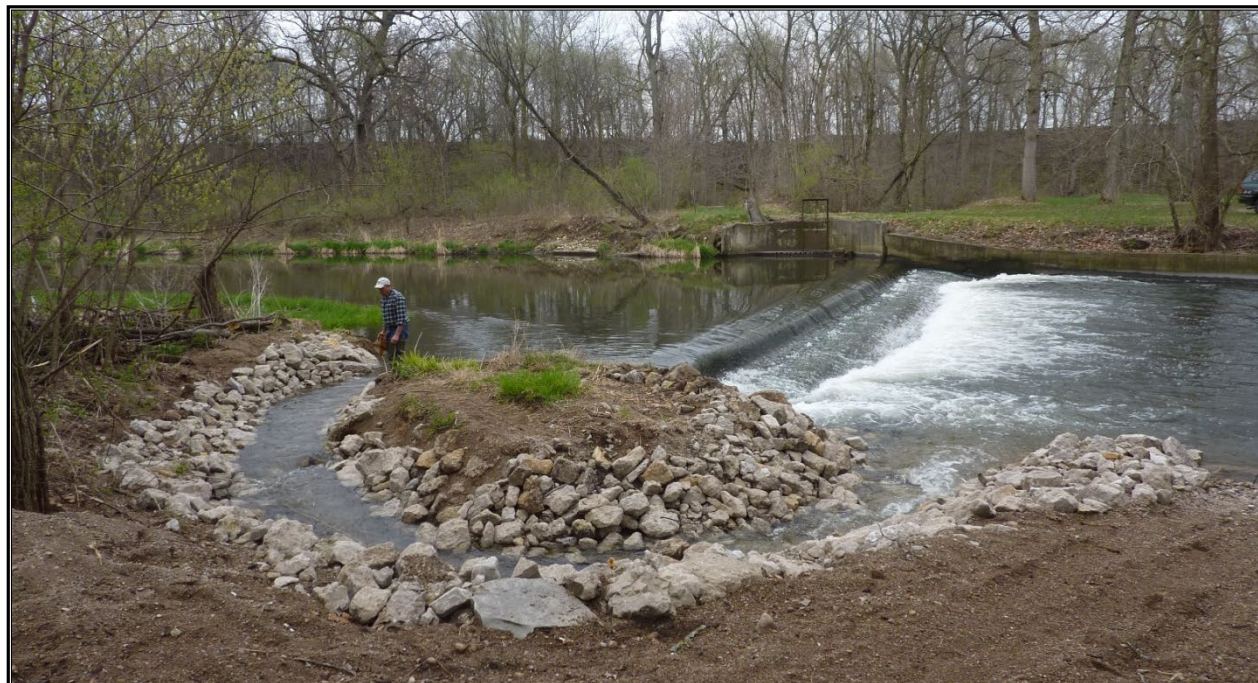
Photo 2: Bypass channel on Big Rock Creek, IL
