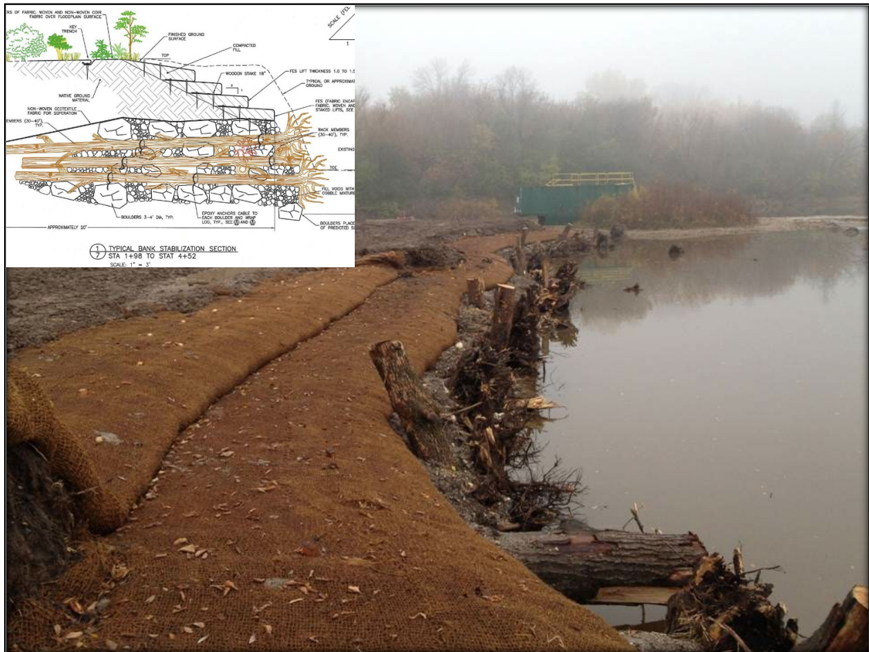
Photo 6: Large woody debris structure and soil terracing
