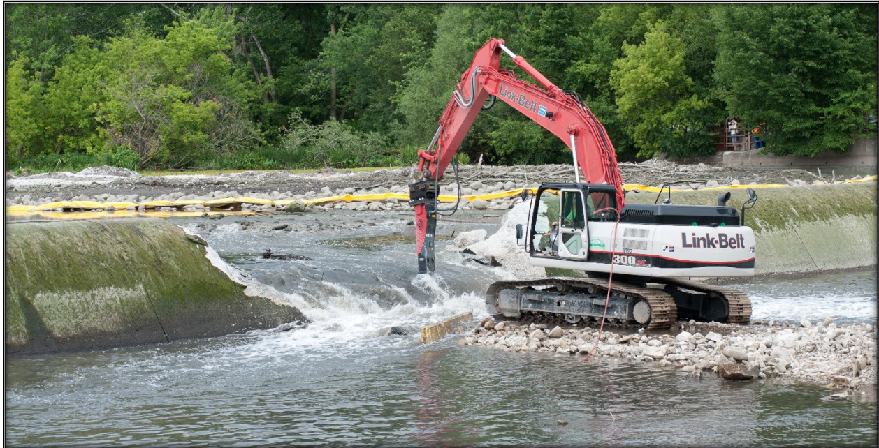
Photo 1: Demolition of the Hofmann Dam, IL
