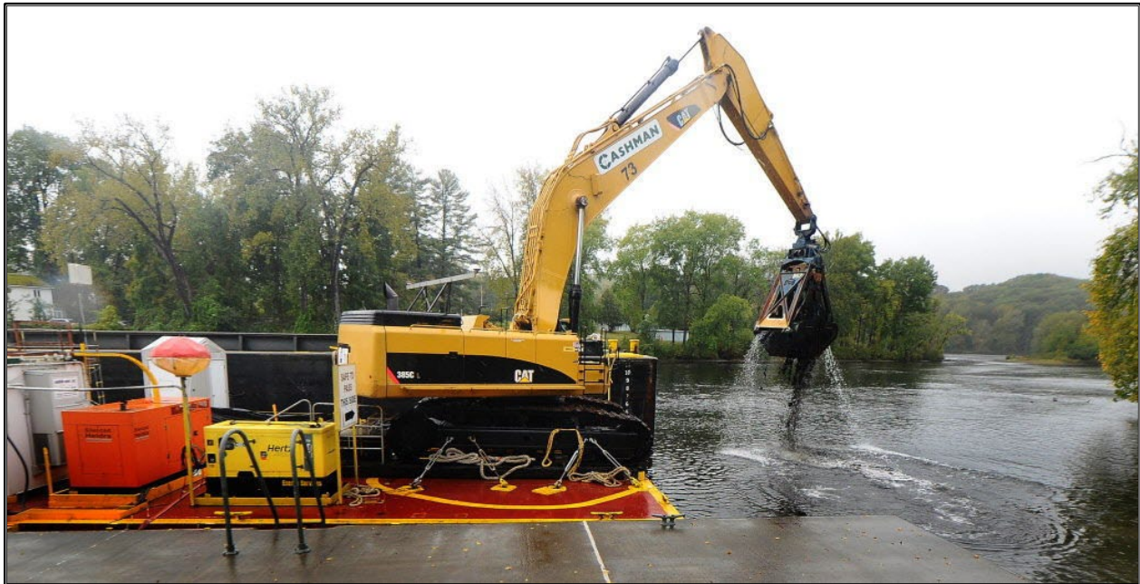
Photo 3: Mechanical riverine dredging of sediments, USEPA
