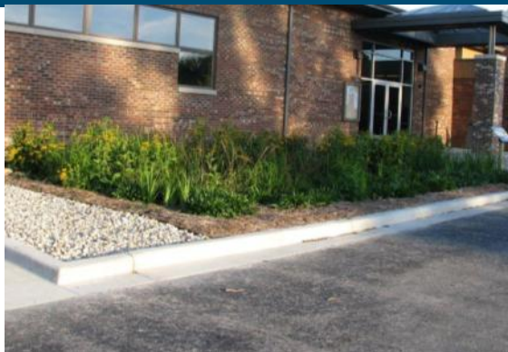
Somers Town Hall rain garden.
