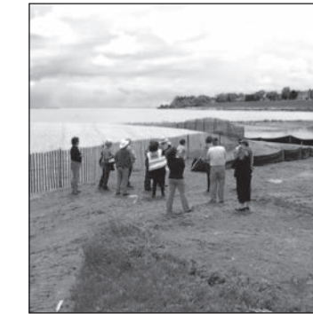
City of Racine's Samuel Myers Park restoration includes dunes and wetlands, native plantings and stormwater features.
