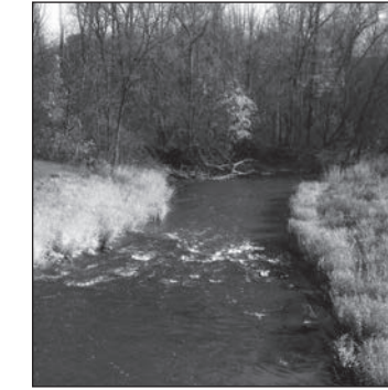
Dam removal and streambank restoration at the Kenosha Country Club spawned new interest in restoring the Pike River
